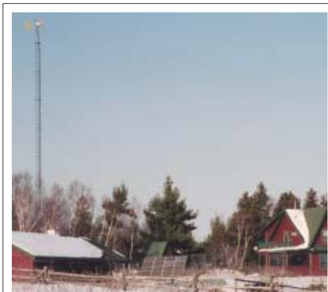
Figure 1. This off grid home is typical of many rural properties, with the exception of the wind turbine, photovoltaic panel and lack of electrical bill.
