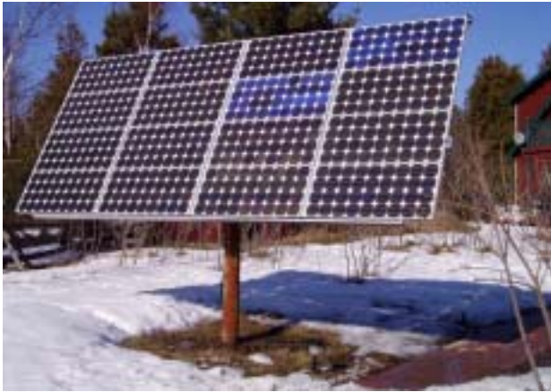
Figure 11 Unlike fossil fuels or nuclear energy, renewable energy sources are just that, renewable. No matter how much sunlight we capture with our photovoltaic panels, there will always be more for everyone else; moreover, we're not dumping today's pollution on tomorrow's children. The photo above shows a 1200-Watt peak-output PV array on a sun tracker mount.
